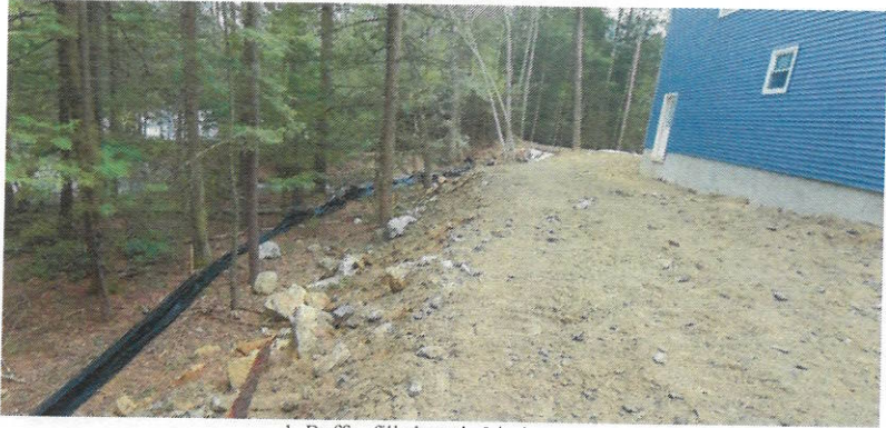
1. Buffer fill slope behind garage
