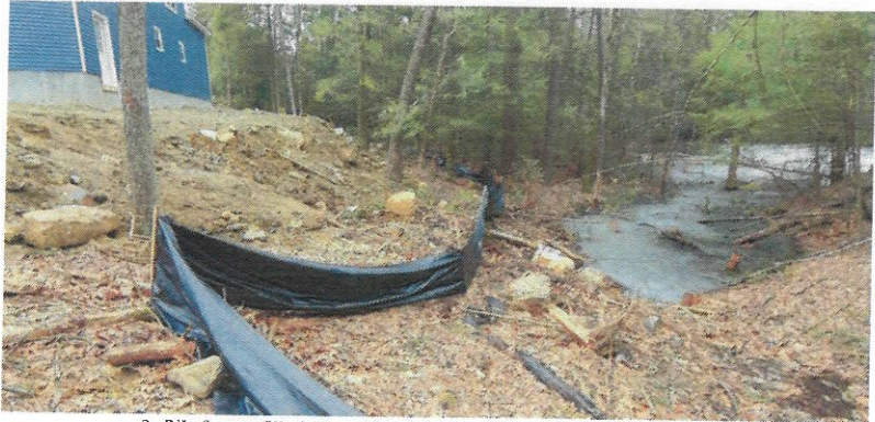
3. Silt fence, fill slope and wetland looking back towards garage
